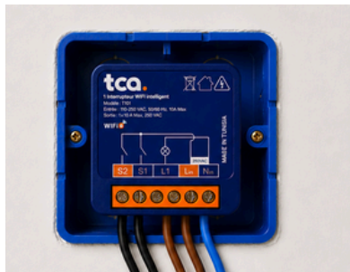
Figure 4: Raccordement du module
